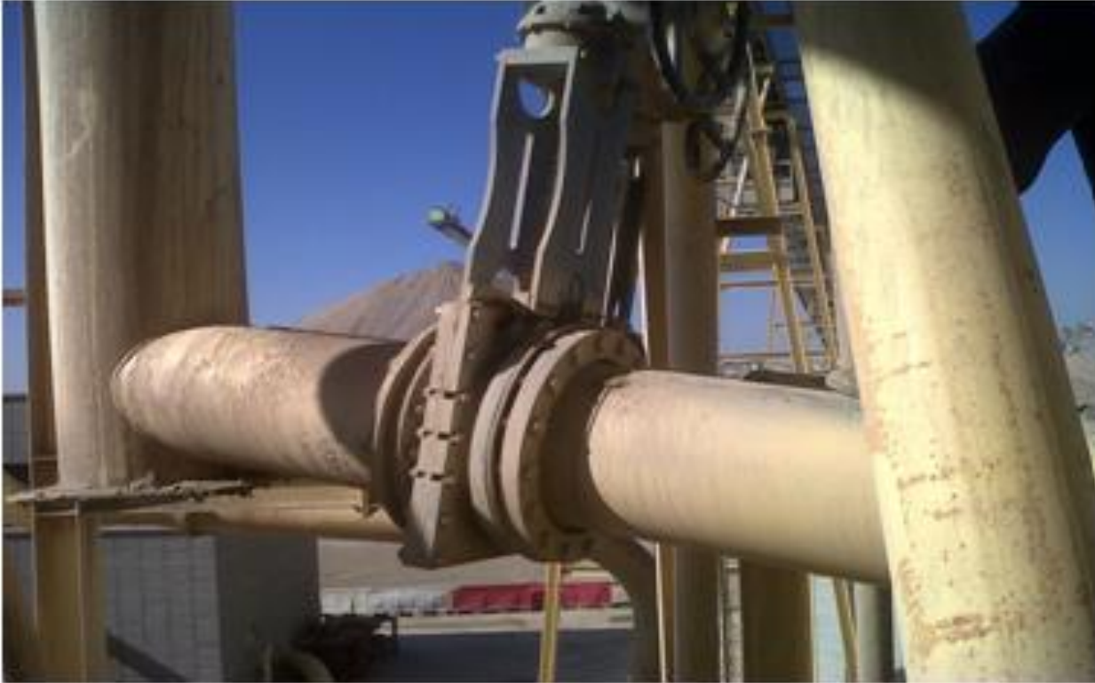
Copper mining, valve DN250, Chile
